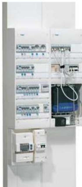
Figure I.10 : Gaine Technique de Logement [7]
