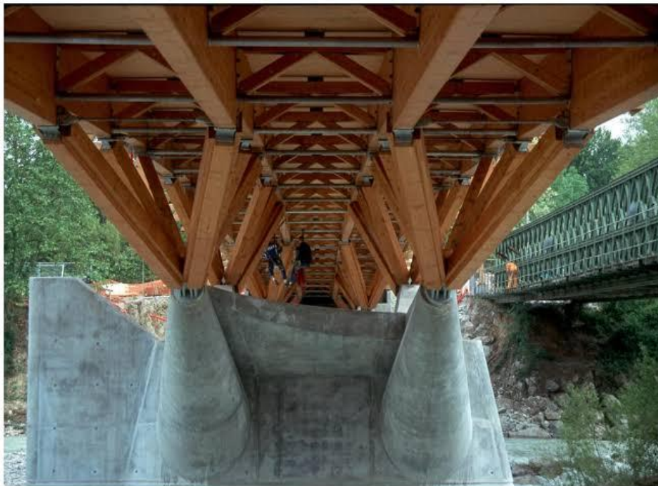
Figure 1-1 Photo illustrant un pont routier [4]
